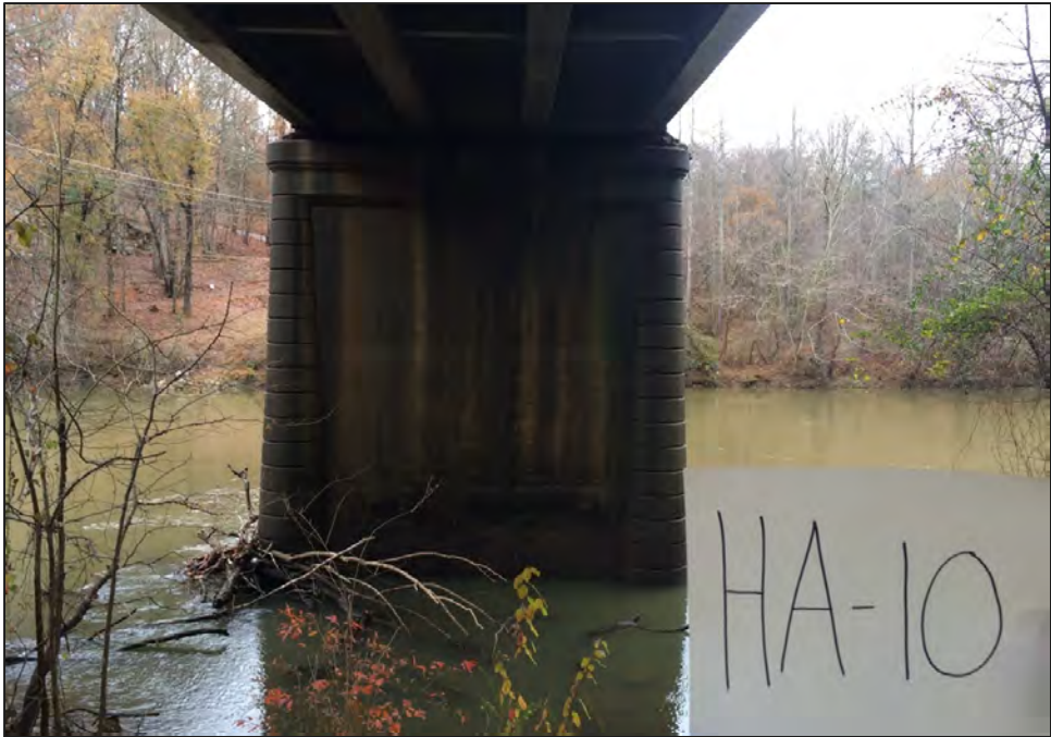
Photo: 10 Date: December 6, 2016 Description: View of pier concrete (HA-10).
